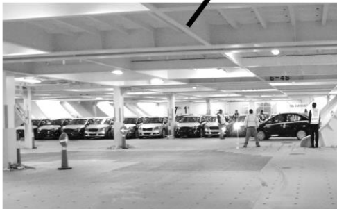
Inside of PCC
